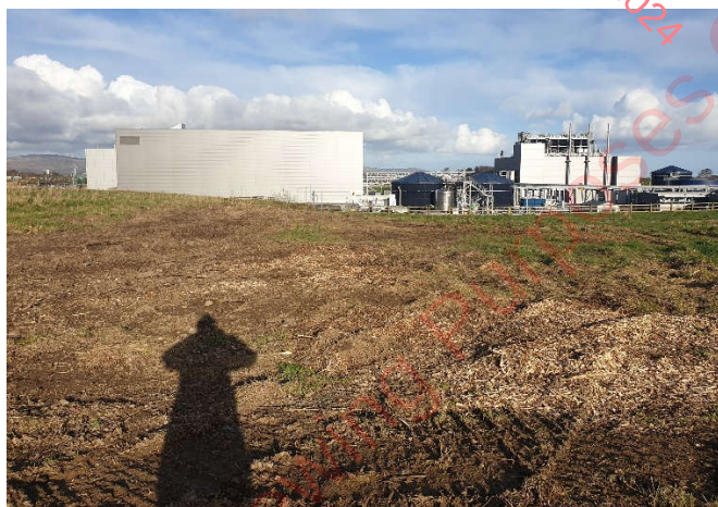
Plate 6-11(b) View northeast of the existing wastewater treatment and main building
