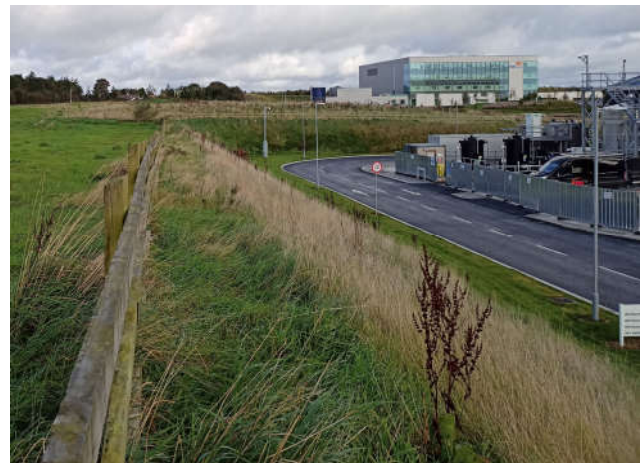
Plate 6-6 Notable drop in elevation from original and the Site existing facility and service road
