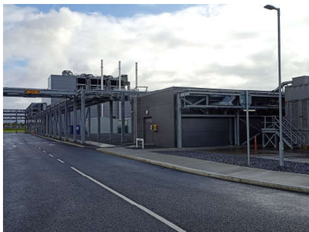
Plate 6-11 (a) Part of the existing wastewater treatment plant
