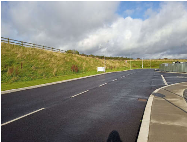
Plate 6-3 Internal access roadway by the Site boundary
